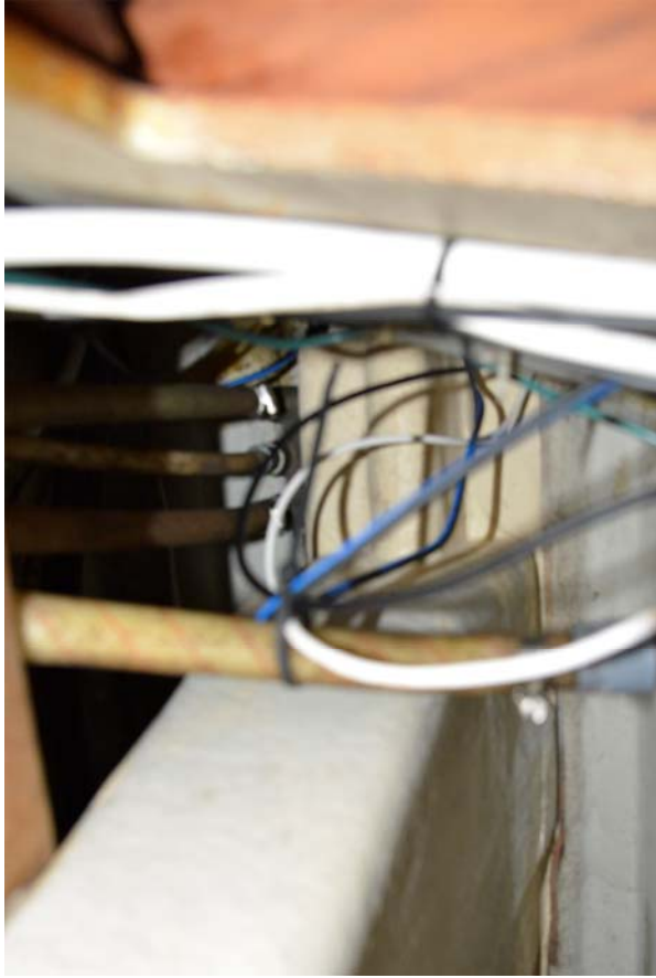
Looking up at the fittings to the deck of the shower.
