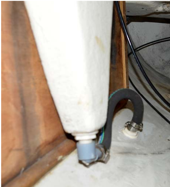
Anchor drain and wooden rode bin to the left.
