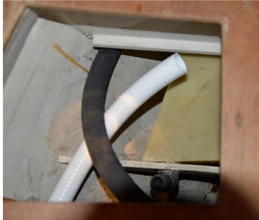
Inspection panel (no screws required) removed. Black is pump-out going to lower/aft/middle of tank. White is new intake (to tank) hose prior to connection.
